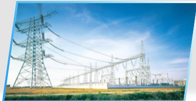
全球电网升级改造 Global Power Grid Renovation and Upgrading
