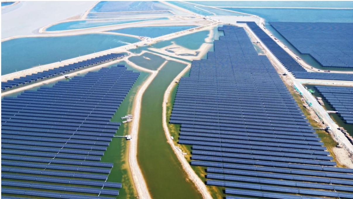
Figure 9.1: aerial view of the Shandong Weiqiao Pioneering 2 GW PV
