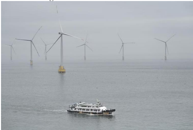
A boat passes wind turbines at the northern end of Pingtan island in south-east China's Fujian province on May 24, 2024. PHOTO: AFP
