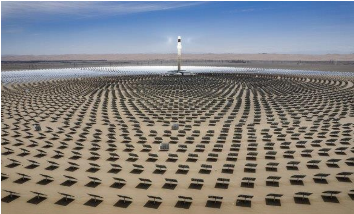
A molten salt tower solar thermal power station in Jiuquan, China.
