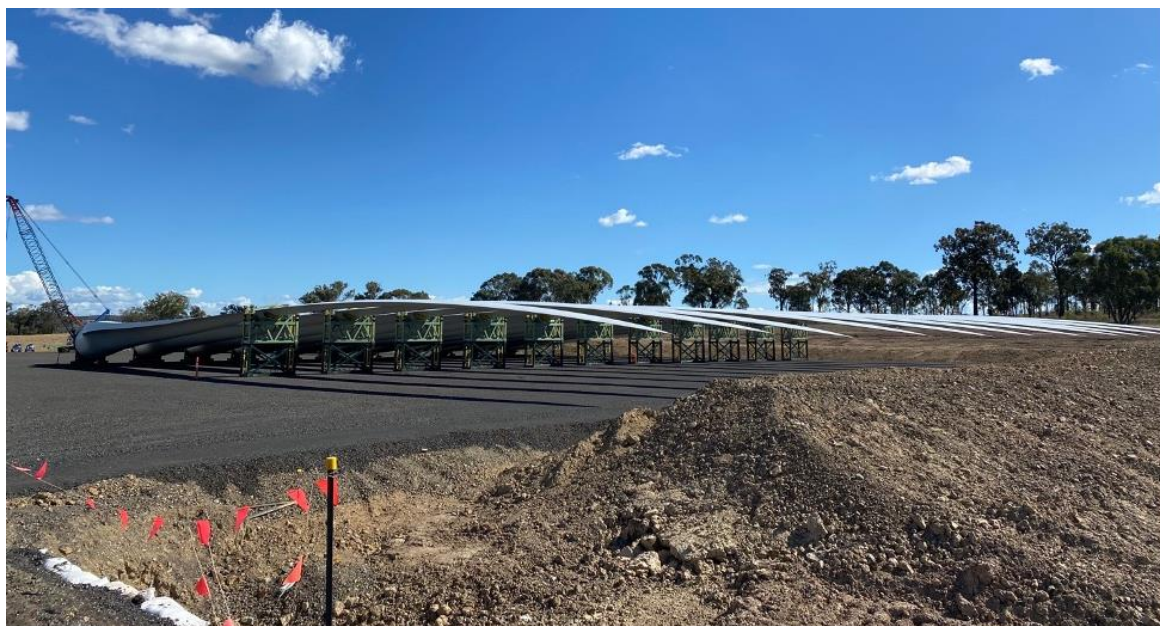
MacIntyre Wind Precinct under construction near Karara, QLD.
