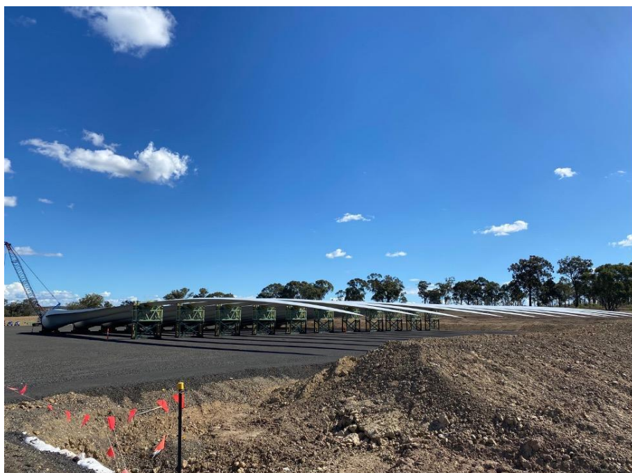
MacIntyre Wind Precinct under construction near Karara, QLD.
